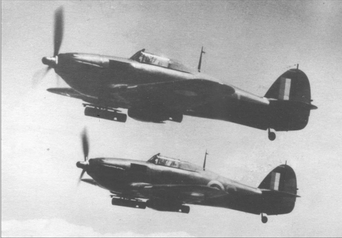
Squadron Hurricanes bombed-up and sporting bedspring bomb racks.
